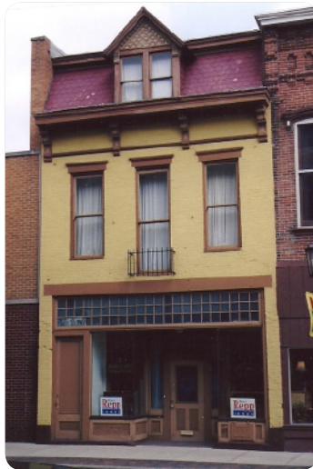
Mansard Roof Addition 1890's. 159 S. Washington Street (photo 2001)
