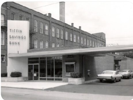
Tiffin Savings Bank 1956. 175 S. Washington Street (photo 1967)
