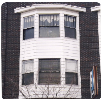
Bay Window. Harding Block 1919. 186-188 S. Washington Street (photo 2001)
