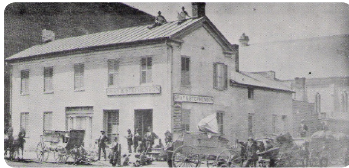
Lugenbeel House 1830. Formerly 154 S. Washington Street (photo c. 1890's)
