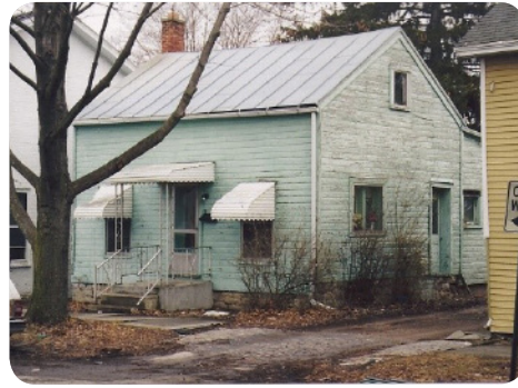
Log House c. 1835. 245 Jefferson Street (photo 2001)
