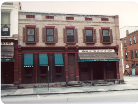
Ebbert House, 64, 66 E. Perry Street Converted to Retail Use in 1886 (photo 1991)
