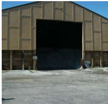
Figure 3-2. Salt storage shed
