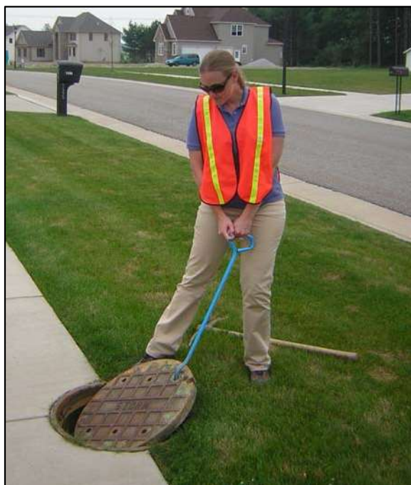
Figure 14: Removing storm drain lid
