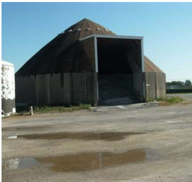
Figure 3-1. Salt storage dome
