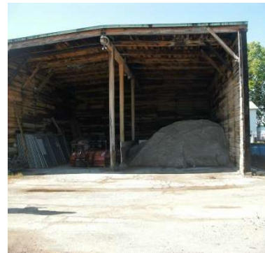
Figure 3-3. Beet juice treated salt covered under storage pole barn
