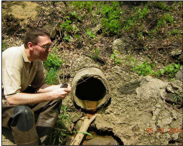
Figure 12: Dry weather field inspection
