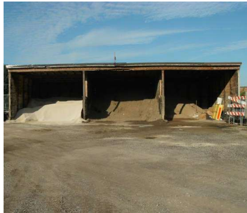
Figure 3-2. Construction materials kept under cover in storage pole barn
