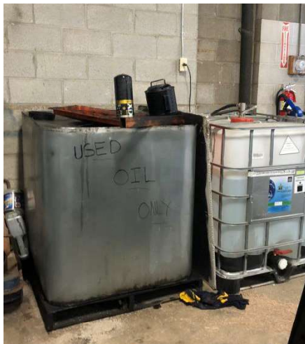
Figure 3-4. Labeled oil totes located inside maintenance garage
