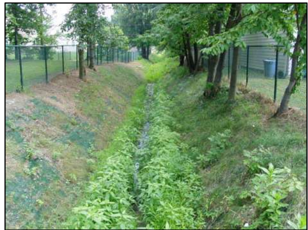
Figure 3: Ditch MS4 outfall
